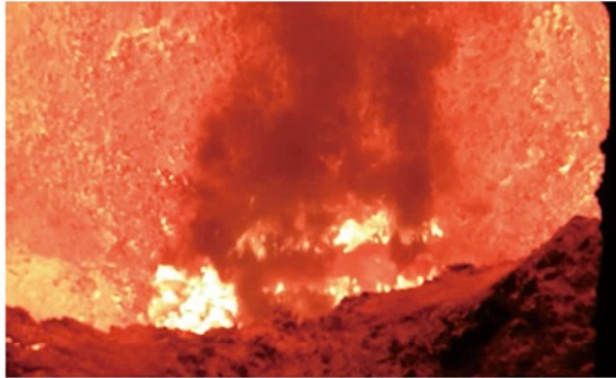
传统大面料烧结20min后依然冒出有毒烟气 Traditional material repairing: still exhaust poisonous smoke after 20min sintering.
