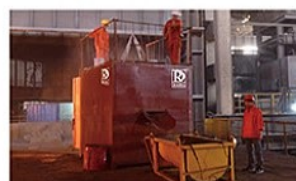
现场搅拌 Site mixing
